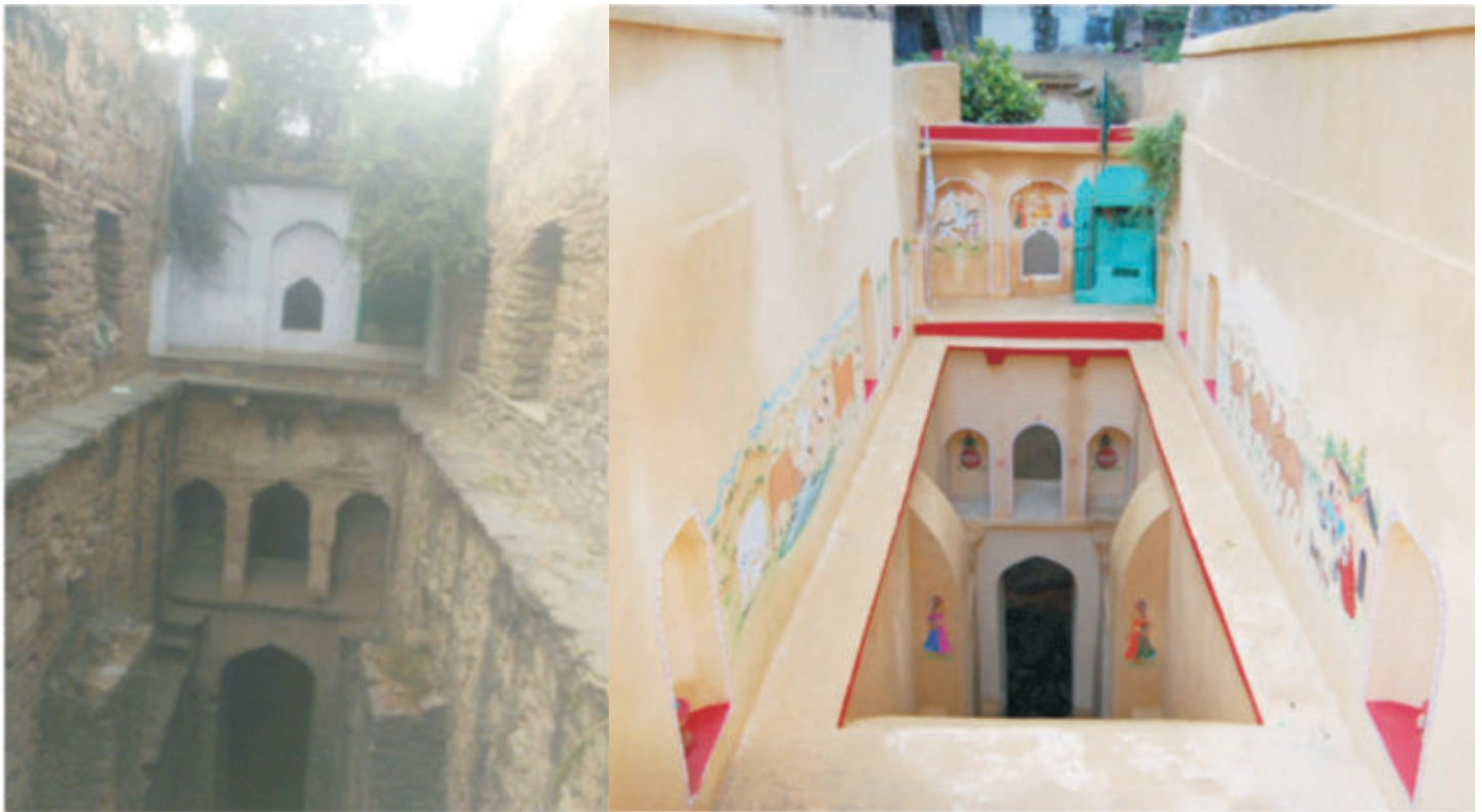
Situation of Sayeed step well before and after Restoration
